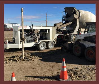
into one hole flows to another hole and pushes the casing out of the ground. This is what happened to the casing in the upper right photo. These holes are sometimes many feet apart.
